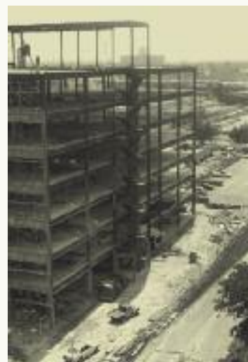
Above: Hofheimer Hall under construction
