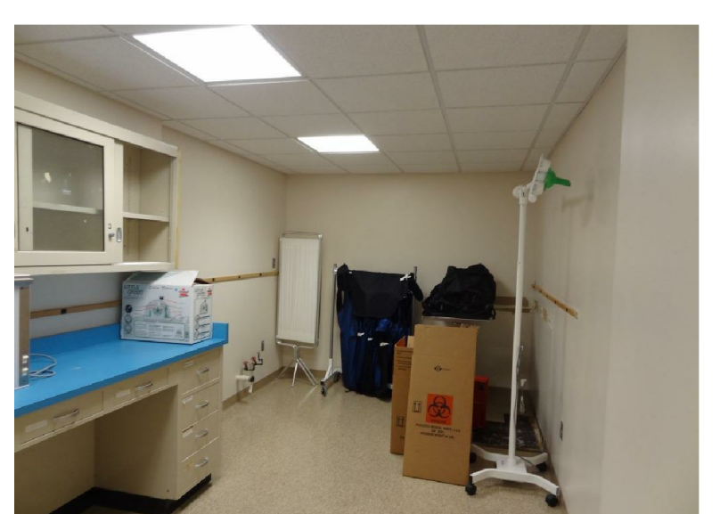
PHOTO #2 - ACM FLOOR TILE AND MASTIC IN ROOM 2064.
